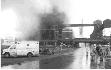
9.2 1999 Ford power plant explosion, Dearborn, Michigan, USA. Courtesy Dearborn Fire Department.
